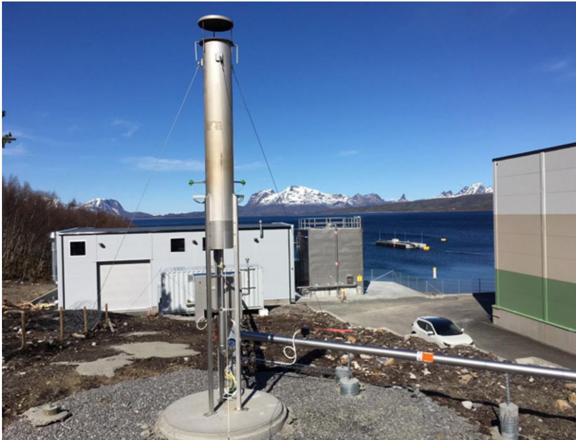
Fig. 8 Forsan plant showing treatment building, ABR reactor, gas storage and flare and part of fish plant
